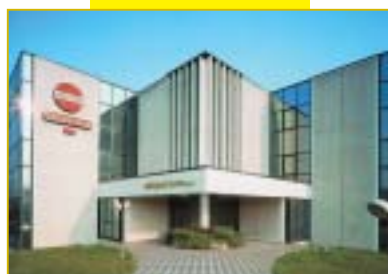
Plant n° 1 - Shrink division - DALMINE
